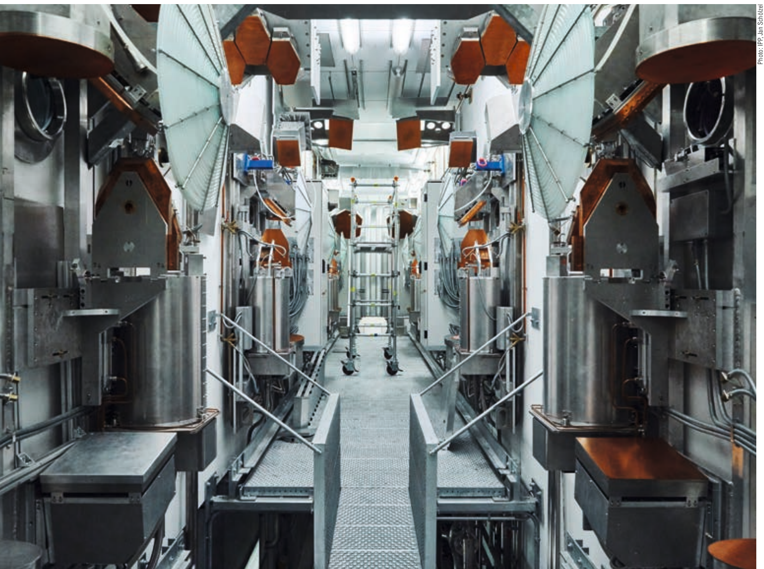
140 metal mirrors transmit the microwaves from up to now ten gyrotrons to the Wendelstein 7-X plasma
