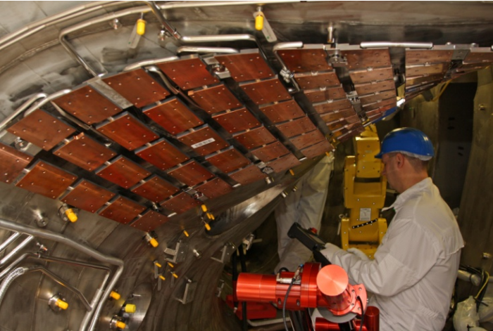
Heat shields in the plasma vessel of Wendelstein 7-X
