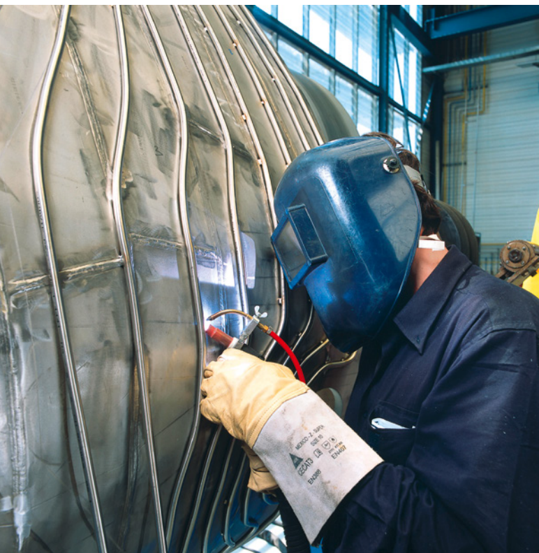
Welding the Wendelstein 7-X plasma vessel
