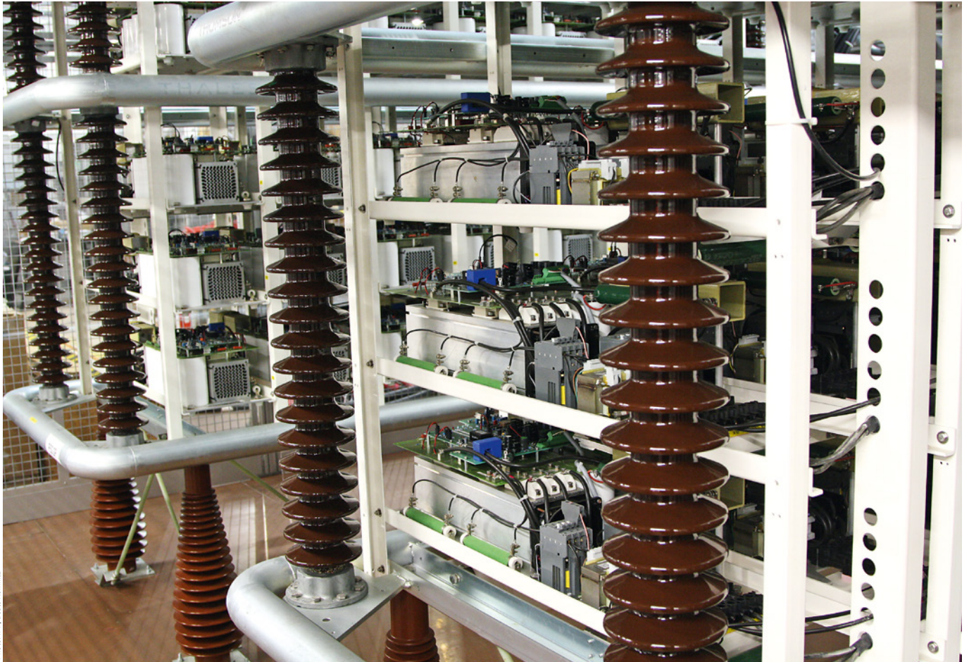
Switching stage racks for the high-voltage DC power system
