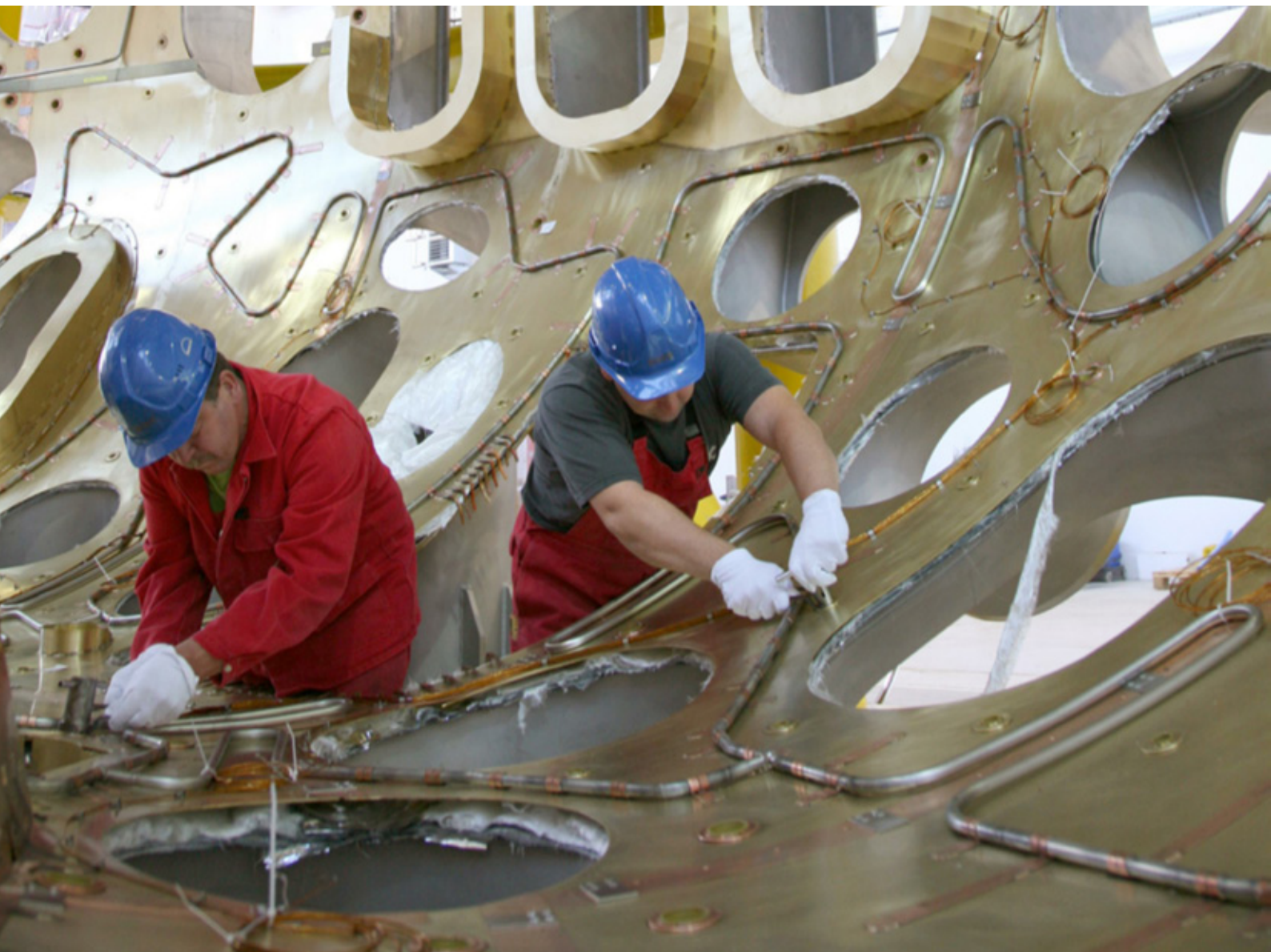
Assembly of the thermal insulation for the outer vessel (brass shields)
