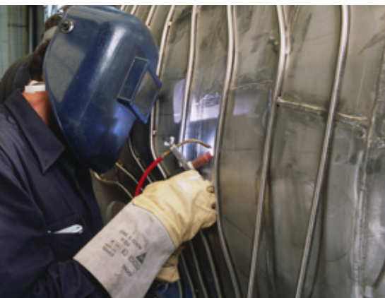
Welding the Wendelstein 7-X plasma vessel
