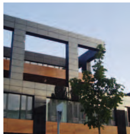
Thin-film modules on a building façade. Helmholtz-Zentrum Berlin
